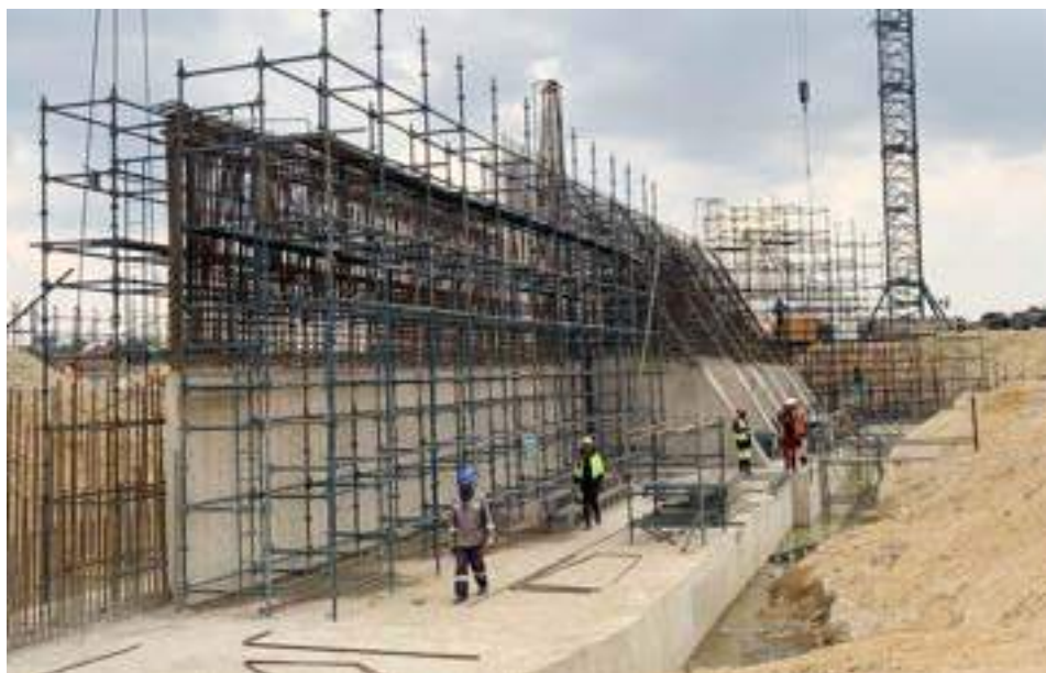
Mbudzi Interchange Construction
