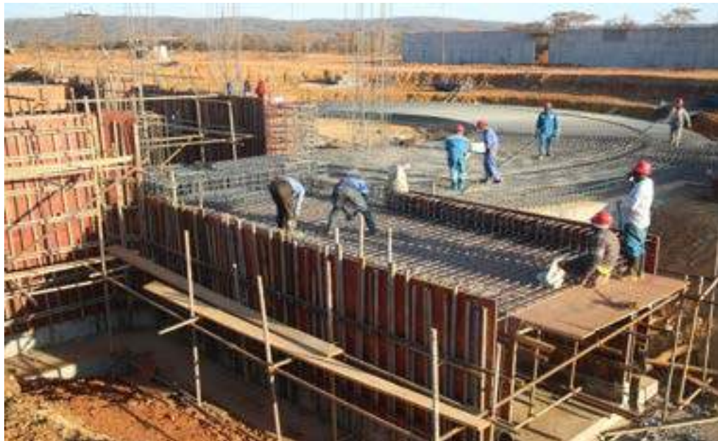
Construction at Manhize
