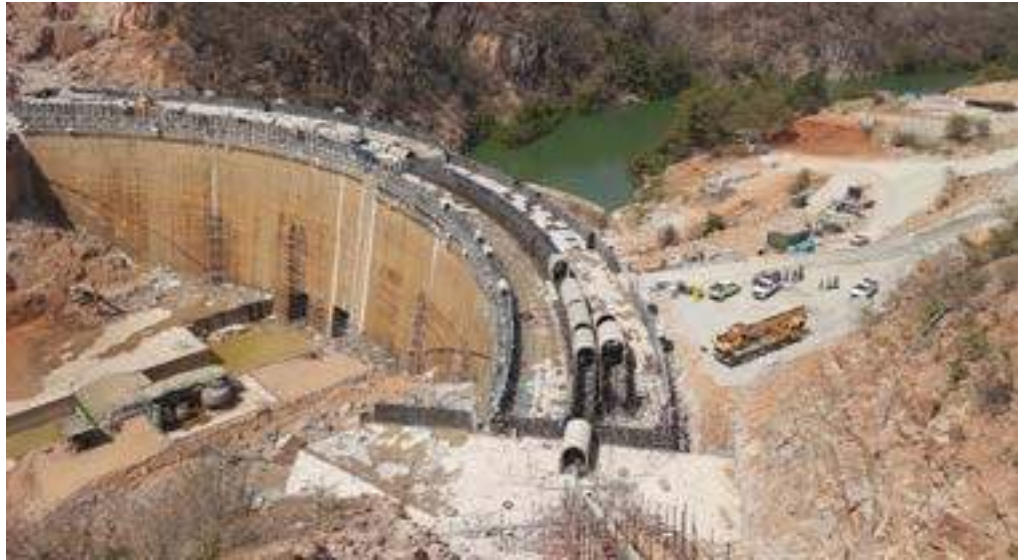
Gwayi Shangani Dam
