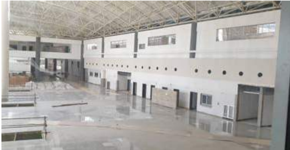
Inside of the Terminal Building
