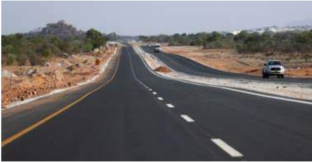
Harare- Masvingo- Beitbridge Road
