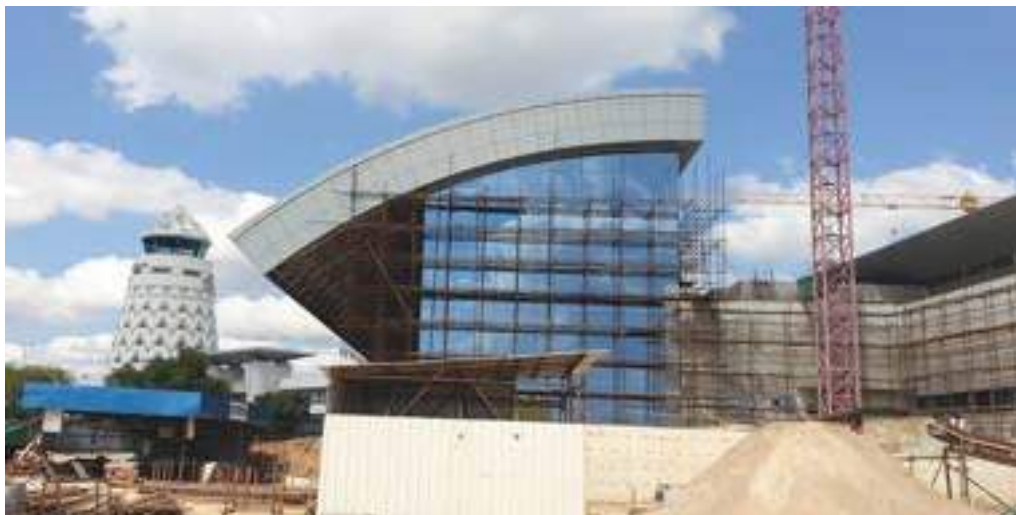
Outside of the Terminal Building
